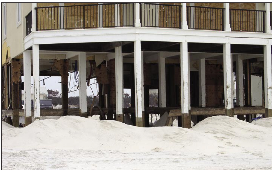
Figure 4: Breakaway walls under an elevated building that were removed by waves (i.e., performed as intended) during Hurricane Ivan in 2004 (Gulf Shores, AL)
